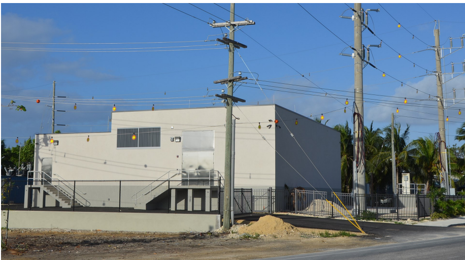
The Prospect Substation was completed in June 2022 and will greatly assist with efficiency in the constantly expanding Prospect area.
